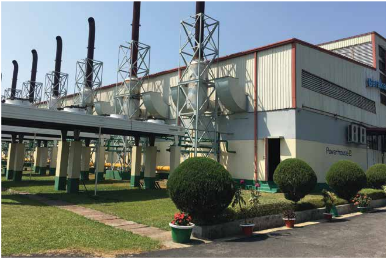
Baraka Power Limited, a concern of Baraka Group, 55.138 MW Power Plant at Fenchuganj, Sylhet, financed by IIDFC.
