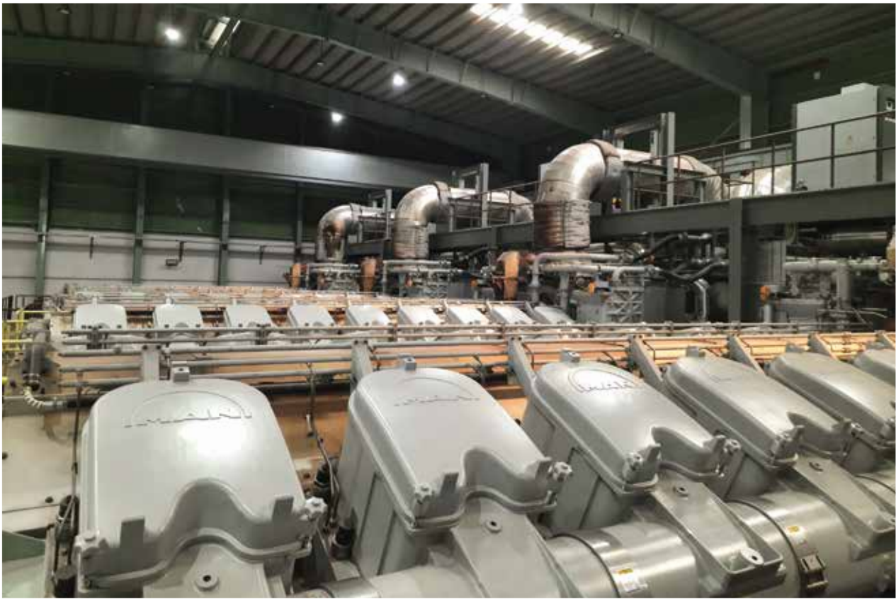
Confidence Power Bogra Limited, a concern of Confidence group, 113 MW power plant project at Birgram, Bogra, financed by IIDFC.
