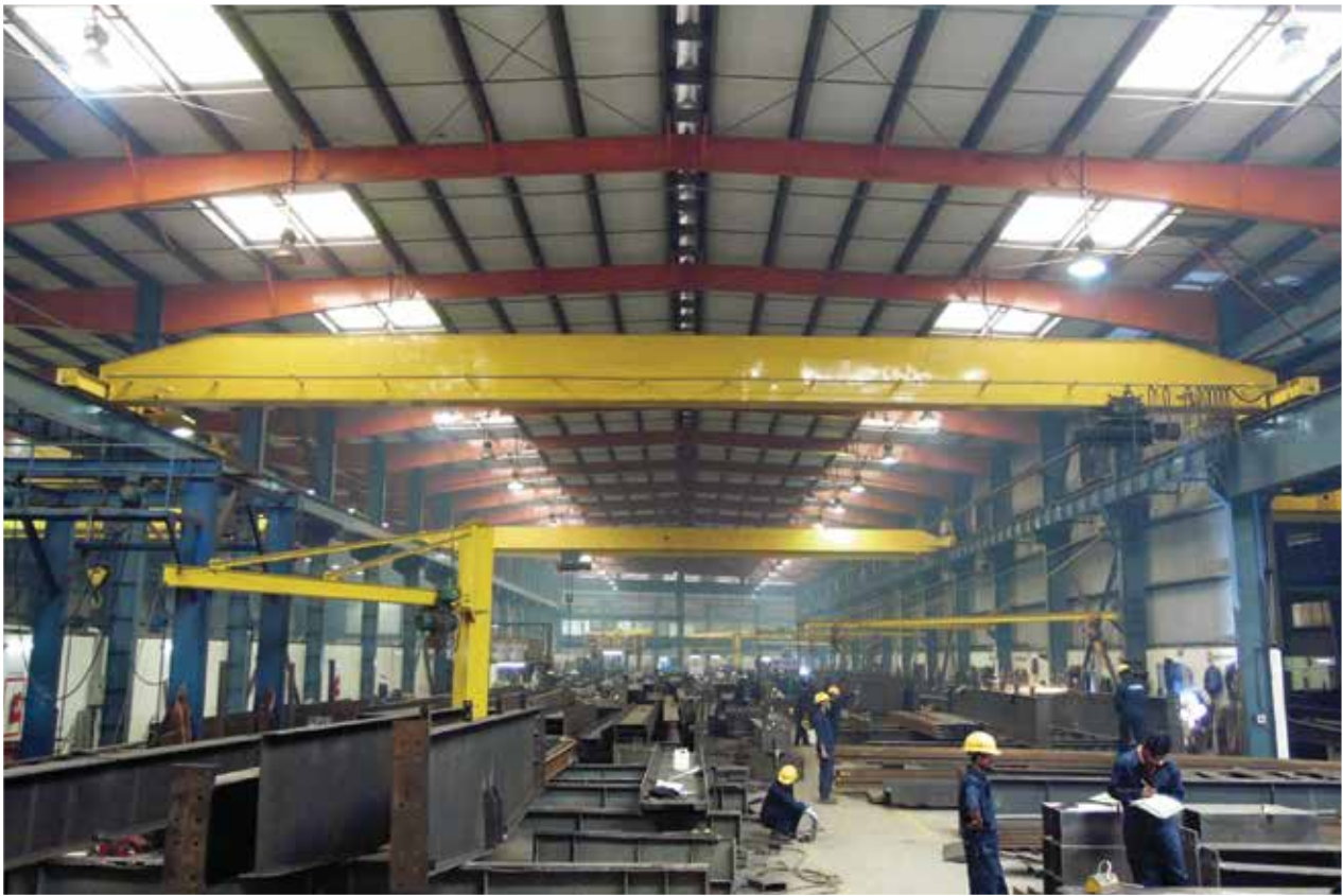
Pre-Engineered Steel Building Manufacturing Company at Chouddagram Cumilla financed under SME.
